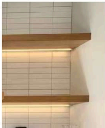
UNDER SHELF LIGHTING IN TALL CABINETS IN CROCKERY/DISPLAY UNIT
